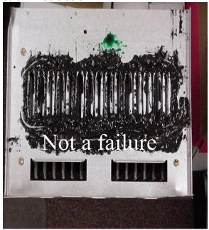
After the heat exchanger is inspected and serviced, re-install the heat exchanger assembly in the furnace. Test the furnace for air leakage around the cell inlet panel area where the heat exchanger assembly attaches to the furnace casing. Seal any air leaks with foil tape or silicone sealant.
