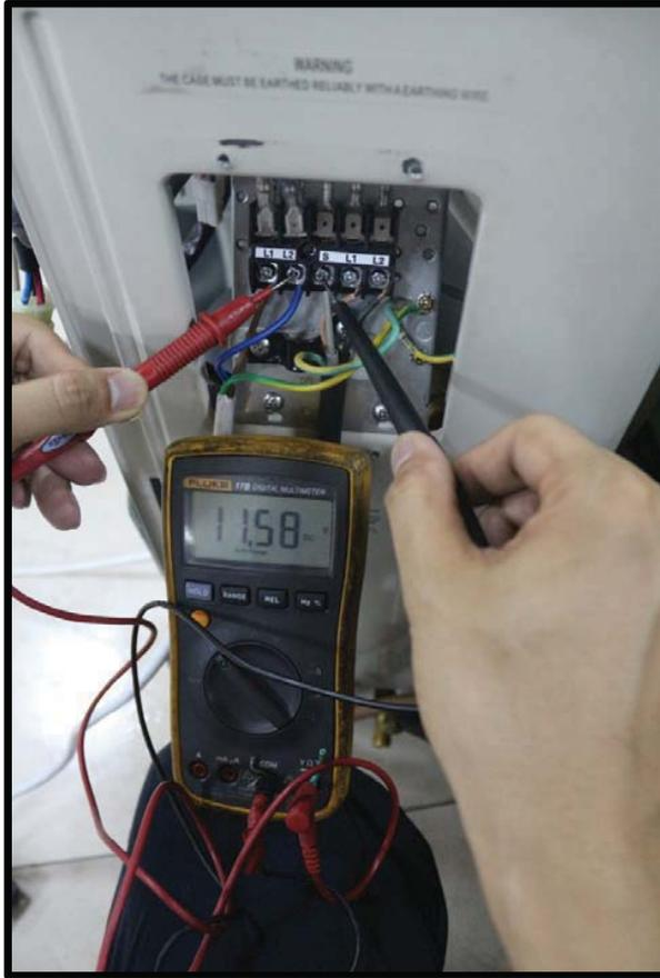
Fig. 29 – Test the DC voltage
